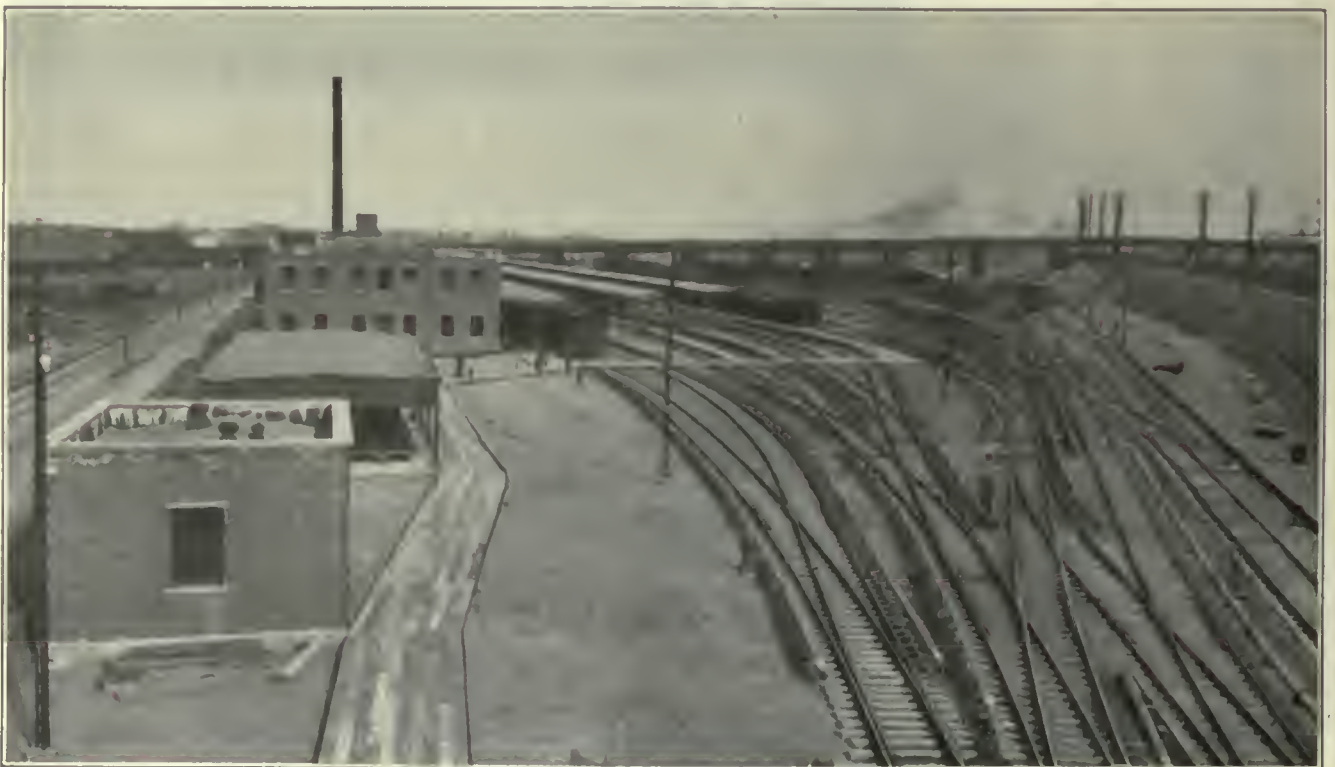
FIG. 509. THIRD RAIL CONTACT SYSTEMS. 600-Volt Over Running Third Rail Construction, Sunnyside Yard, Pennsylvania Railroad, Long Island City, N. Y.
